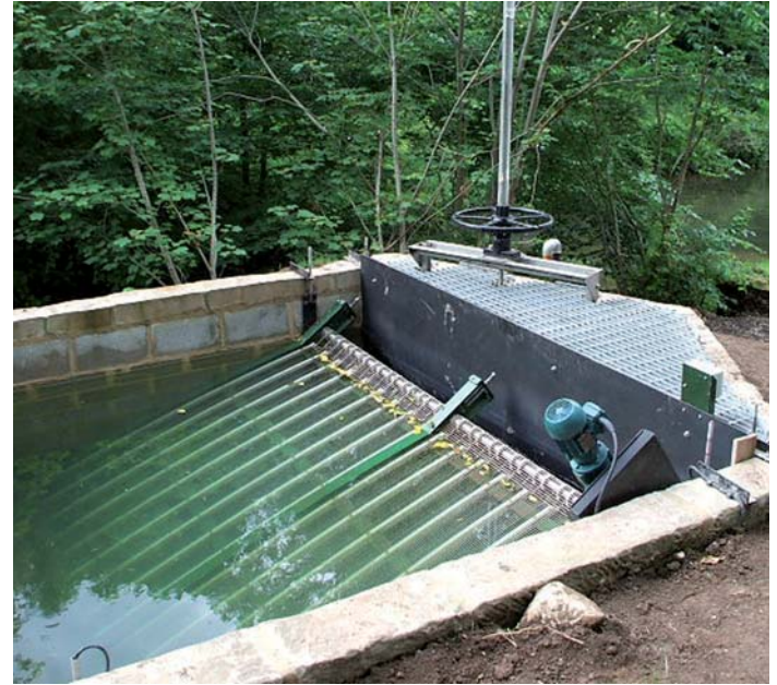
Newly installed band screen at Alport Mill (photo: Derwent Hydro)
