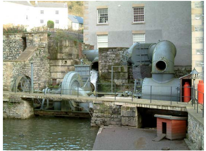
Disused turbines at Cressbrook Mill (Pelton on left; crossflow on right)
