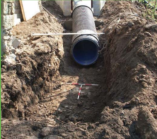
Burying the pipe ('penstock') carrying the water from the intake to the powerhouse at Alport Mill (photo: DHP)
